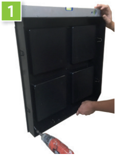
▪ Attach back frame to wall
